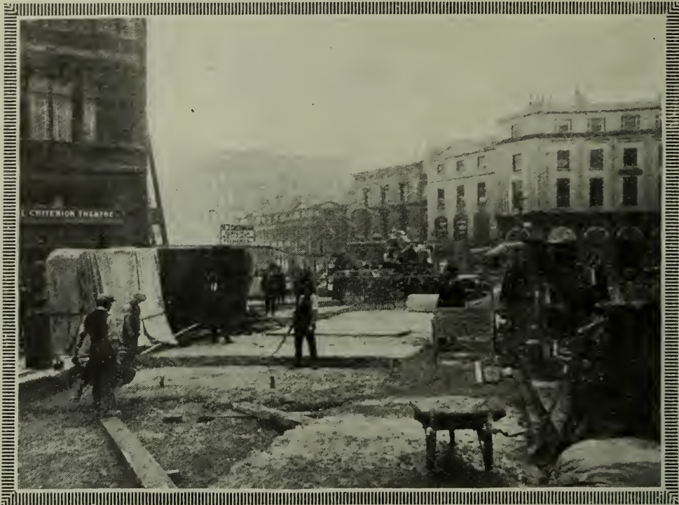
Piccadilly Circus, London. For Westminster Metropolitan Borough. Acting Borough Engineer: L. J. Veit, Esq. Wood Blocks on B.R.C. Foundation.
